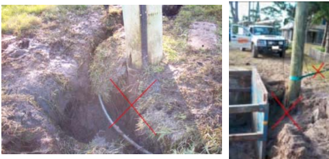
Above: Poles with become unstable if undermined
